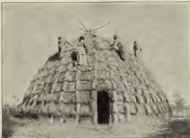
WICHITA GRASS HOUSE IN PROCESS OF CONSTRUCTION. (MOONEY)
